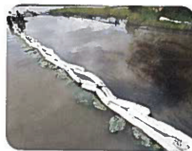
Figure 1 This floating boom has trapped most of the spilled oil.
