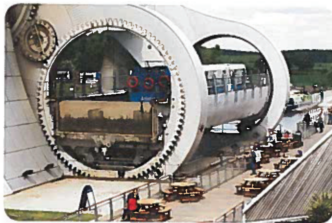
Figure 3 The small gear between the two large ones causes the large gears to turn in opposite directions.
