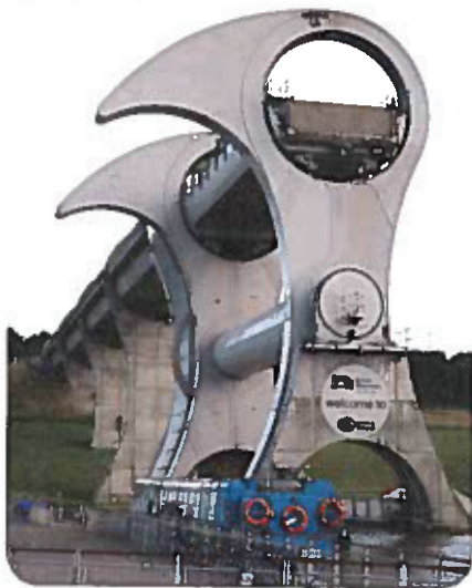
Figure 1 This amazing structure stands more than eight stories tall with a huge tank at the end of each of its two giant arms.
